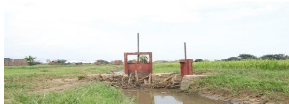
Figure 2 Reality on the ground: Failed Canal system in Burundi
